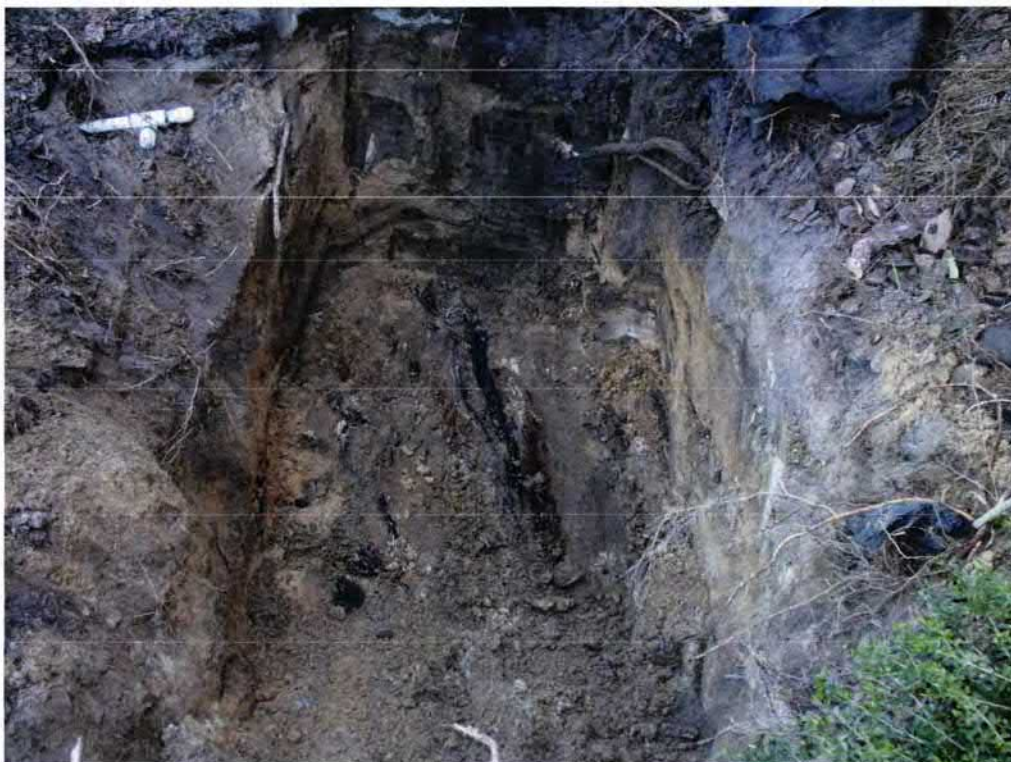
Picture 2: UST 776LaurelBB excavation in progress.
